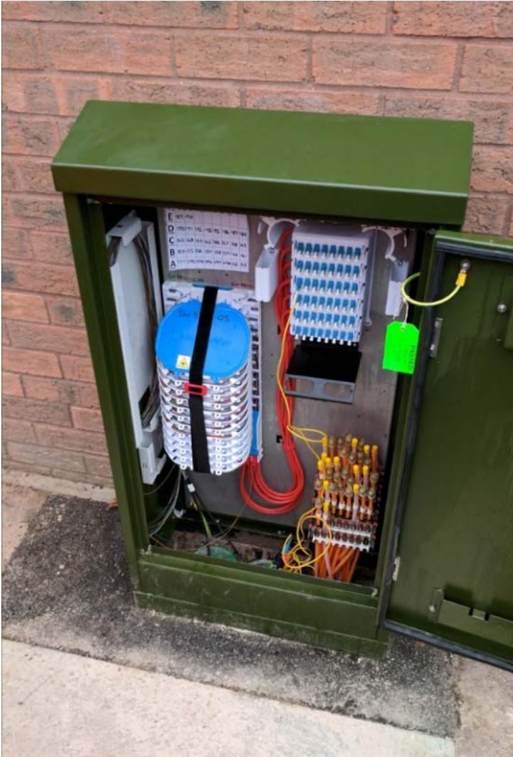
The drop cabinet is the local 'street' fibre patch cabinet and is now installed to support the new microduct based delivery (it was not required when Gigaclear used to direct bury the access fibres). It is a passive cabinet and typically holds up to 48 property specific micro ducts, allowing the fibres inside to be patched into the local access cabinet.
